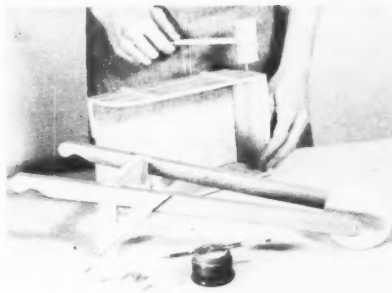
Apply glue to the hardwood pegs before driving them home. Space nails to avoid the pegs.
